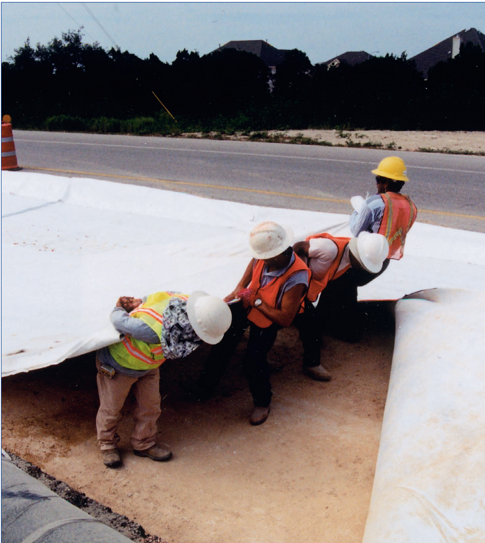
Maine U.S. Route 1, Roadrain for subsurface drainage. MN Steele County Highway 35, Roadrain for capillary break layer. Texas, Austin Southwest Parkway Roadrain for seepage water interception.
