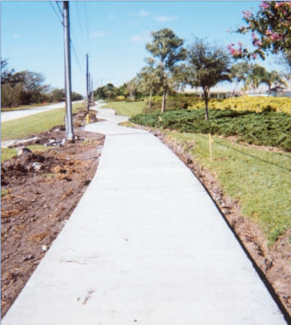
Rock-in-Roll under sidewalk in Florida.
