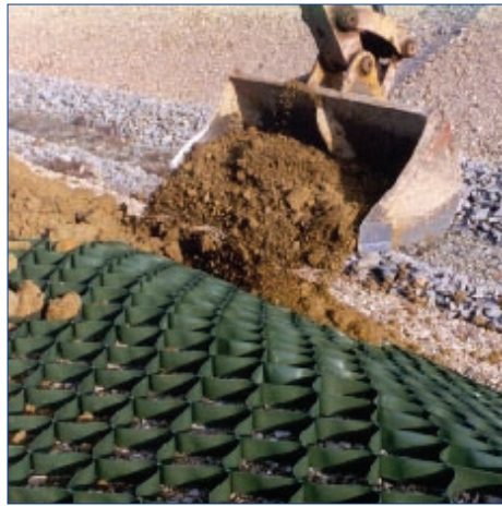
Tenax Multimatt 100 TRM for park farm drainage, UK. Tenax Tenweb 300 cellular confinement system for slope erosion control, New Mexico. Tenax Silt Fence for sediment control, Maryland.
