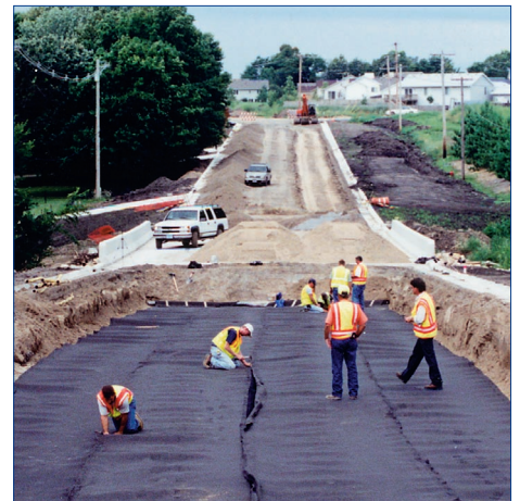
Maine U.S. Route 1, Roadrain for subsurface drainage. MN Steele County Highway 35, Roadrain for capillary break layer. Texas, Austin Southwest Parkway Roadrain for seepage water interception.
