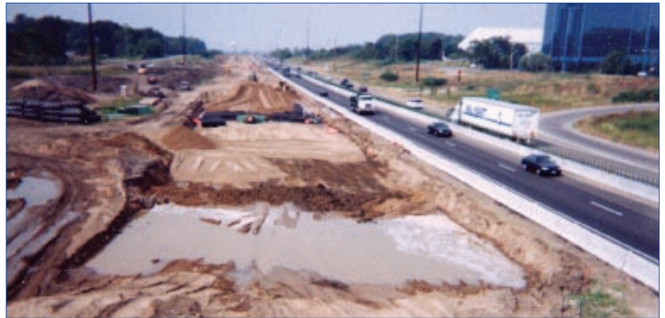
Standing water in a highway during construction. Tenax Roadrain for pavement Drainage on VA Route 58, Virginia.
