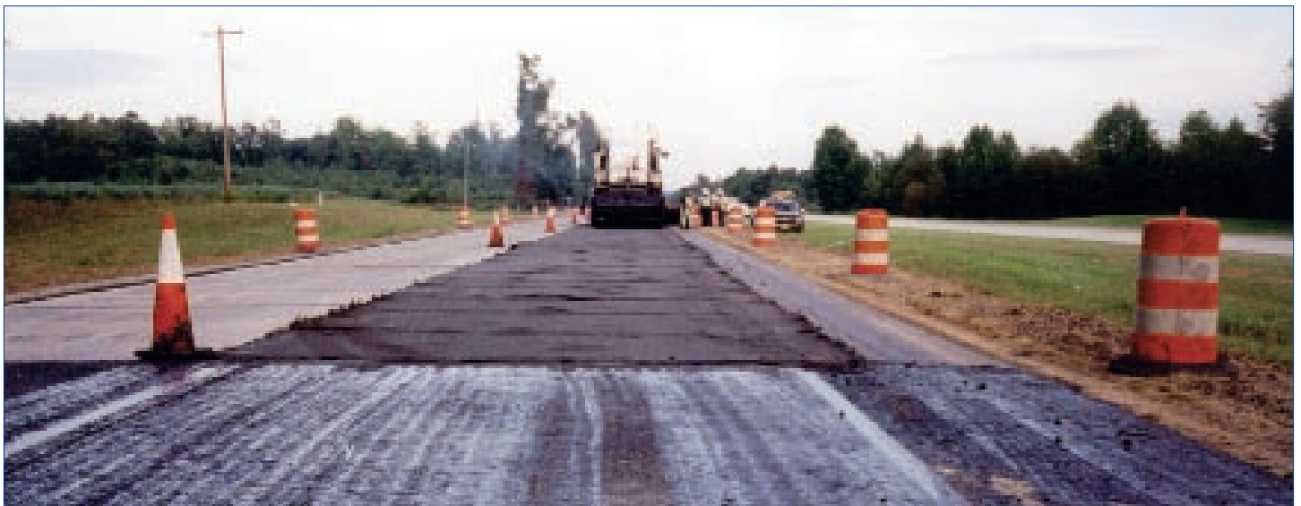
Standing water in a highway during construction. Tenax Roadrain for pavement Drainage on VA Route 58, Virginia.
