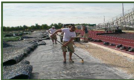
Perimeter trench placed under the Sport Drain Max, Schertz Cibolo ISD, TX.
