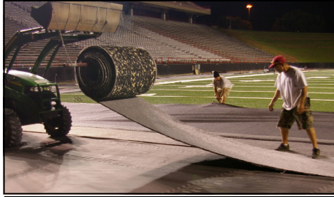
Installation of SDM at the University of Louisiana—Lafayette (Cajun Field 2008)
